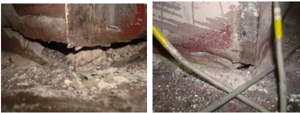
Figure 10: Fracture of west column (Northwest Corner) at 2.3% drift.
