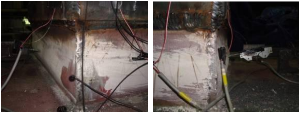
Figure 9: Local buckling of west column (West Side) at 1.8% drift.
